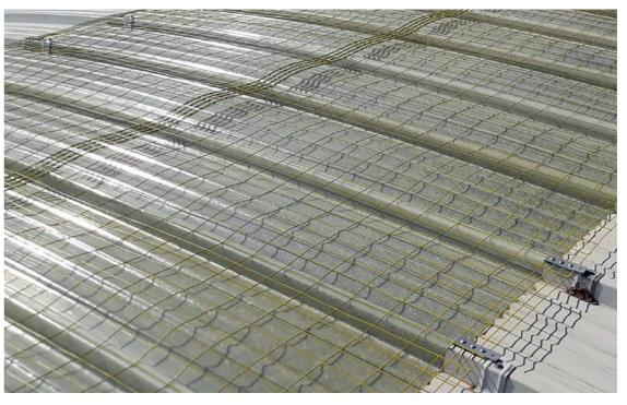
Thanks to its particular coating, the SAFETY NET HI-VIS 600-1200J is ideal for protecting horizontal light points in industrial environments and can be positioned both above and below the covering layer and also in outdoor environments classified C-5 for corrosivity, yellow color as per Legislative Decree n. 81.
