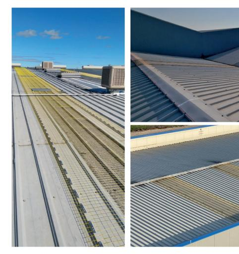
Pasini SAFETY SYSTEM, an articulated and complete range of permanent antifall systems and all the accessories that are necessary for their installation: a line of products - certified according to the regulations in force - aimed at protecting workers from the risks of falling during the installation and maintenance of buildings covers.
